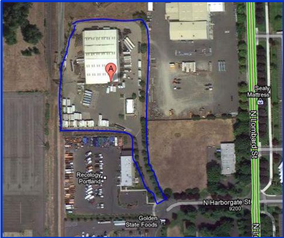
Aerial View of the Portland, OR Processing Facility. 5.11 Acres
