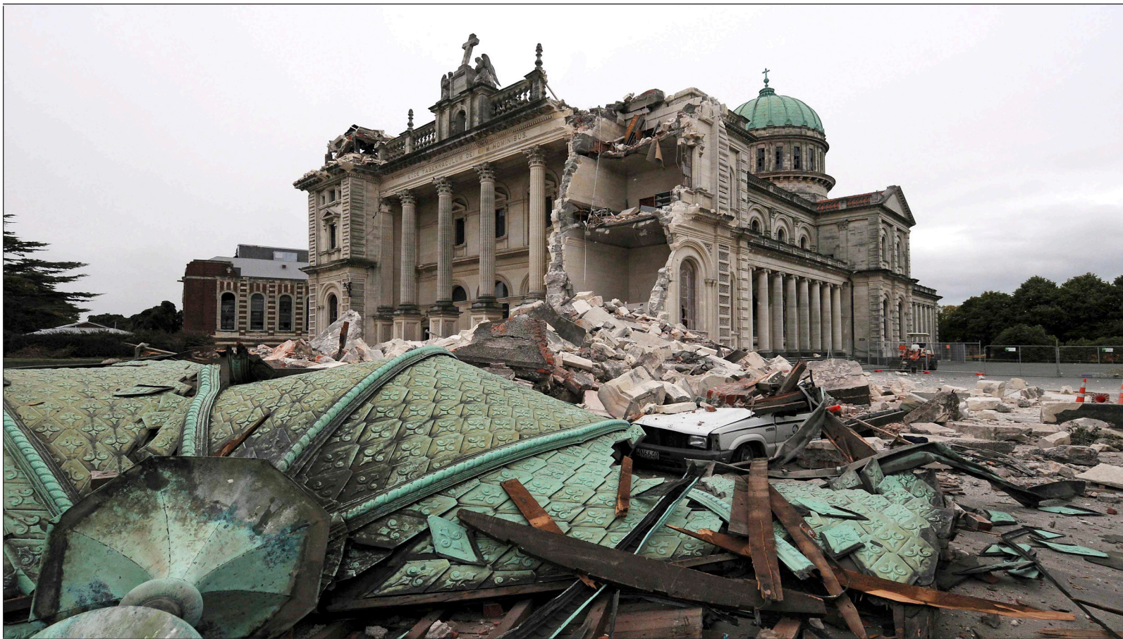
Left: Debris crush a car outside the Christchurch Catholic Cathedral after an earthquake rocked Christchurch, New Zealand, Tuesday, Feb. 22, 2011. The 6.3-magnitude quake toppled tall buildings and churches.
